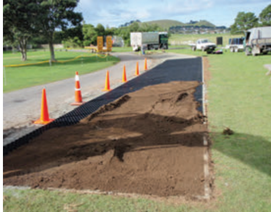
1. Laying of JakMat in May 09
